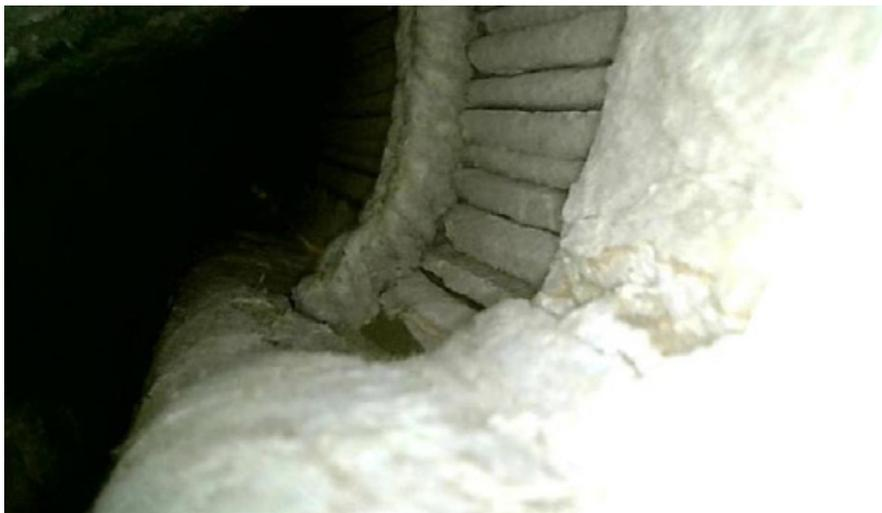
**Fig. 3.** Inspection of the sewing structure under the cover with a probe.
