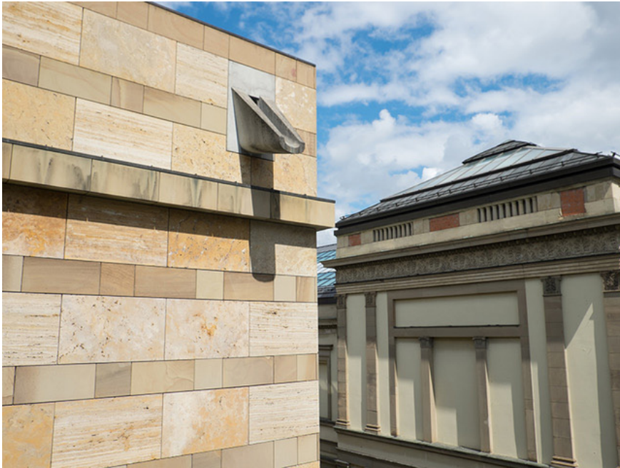
Fig. 1. The Staatsgalerie in Stuttgart: Stirling's elevation towards the old building.
